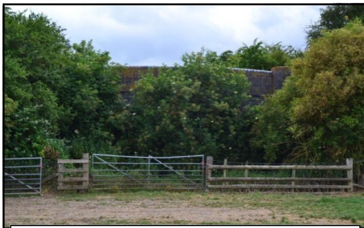
Bridge 14, taken in 2017, looking west. thanks to Simon Stevens, taken from the SMJ website
